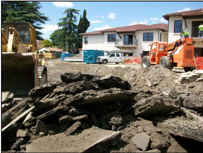
Above: Large pieces of asphalt are lifted off Plymouth Road to make room for a pedestrian walkway. Below: The view from New Merritt shows Norton Garden and the future native plant garden and pathway between the buildings.
